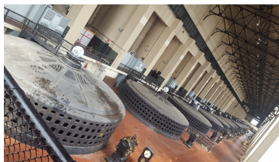
A series of Generators at Ameren Missouri’s Hydroelectric Generating Facility on the Upper Mississippi River near Keokuk, Iowa.
